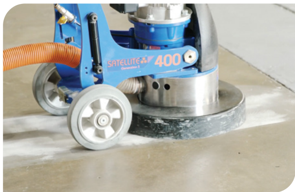
Mechanical abrasion of concrete surface.
