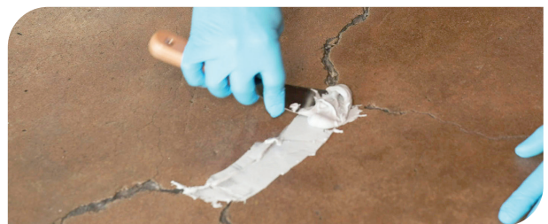
Work the Megapoxy P1 into the crack.
