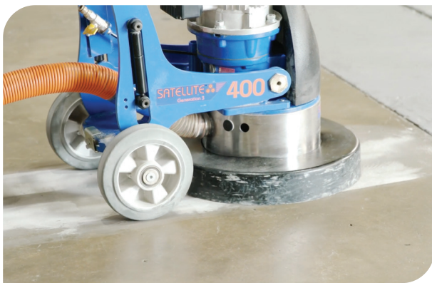
Mechanical abrasion of concrete surface.
