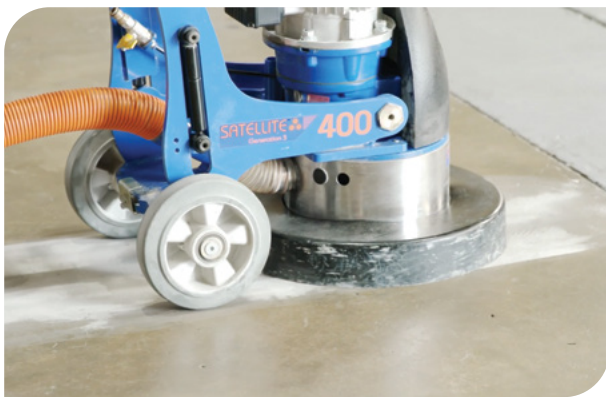
Mechanical abrasion of concrete surface.
