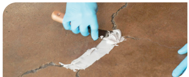
Work the Megapoxy P1 into the crack.
