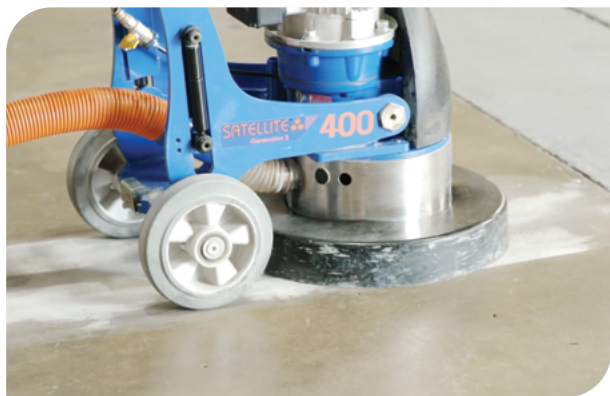
Mechanical abrasion of concrete surface.
