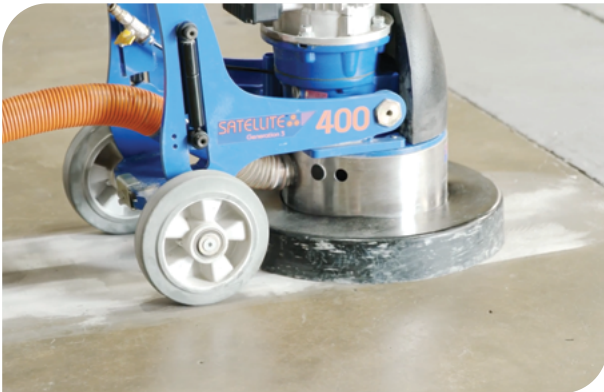
Mechanical abrasion of concrete surface.
