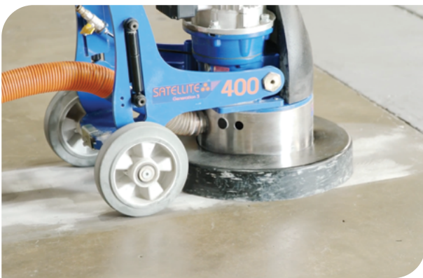
Mechanical abrasion of concrete surface.
