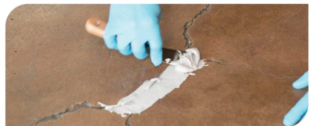
Work the Megapoxy P1 into the crack.
