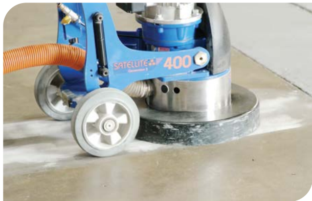
Mechanical abrasion of concrete surface.
