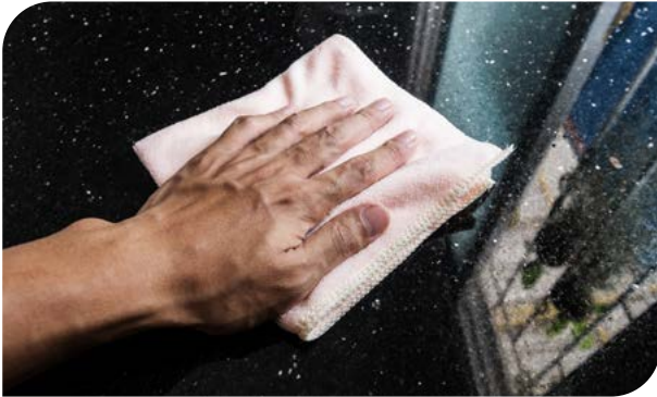
Marble and granite panel surfaces must be clean and dry.
