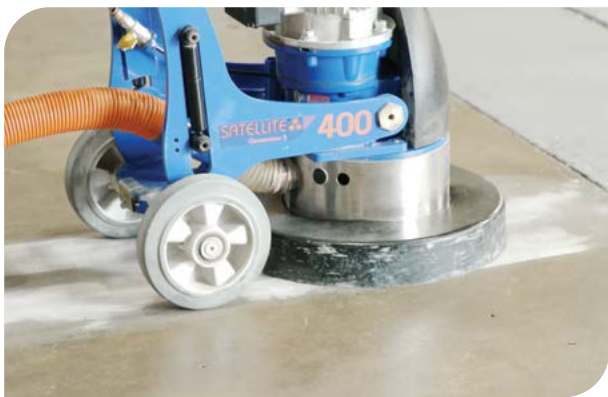
Mechanical abrasion of concrete surface.
