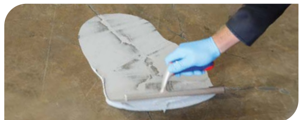
A small amount of moisture on a trowel will allow the surface to be finished smoothly. Re-wet tool frequently to prevent dragging.
