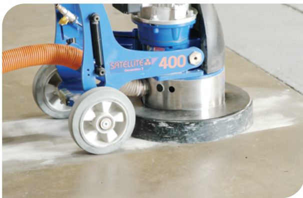
Mechanical abrasion of concrete surface.
